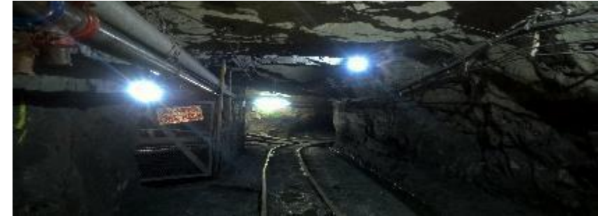
Underground Development drives
